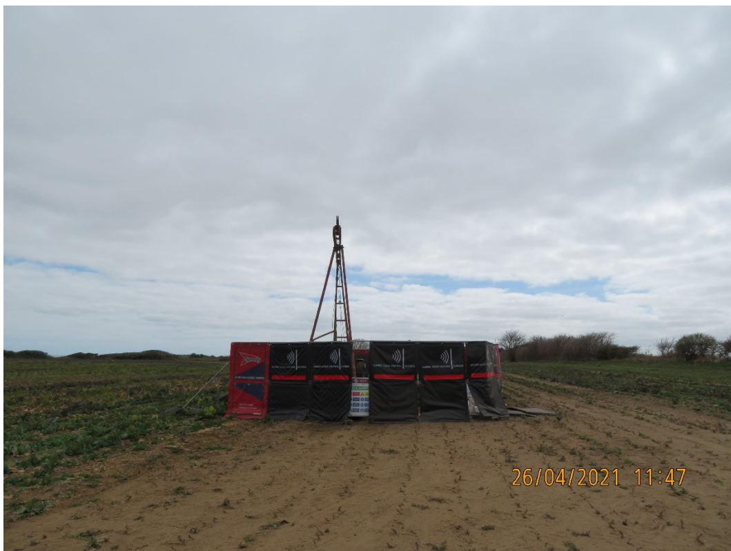
Plate 2.3: Cable Percussion Drilling Rig Compound at the Landfall (with Acoustic fencing)
