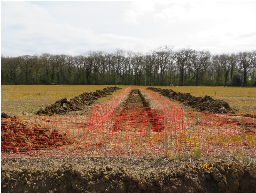
Plate 2.5: Trial Trench Excavated at the Onshore Substation Location
