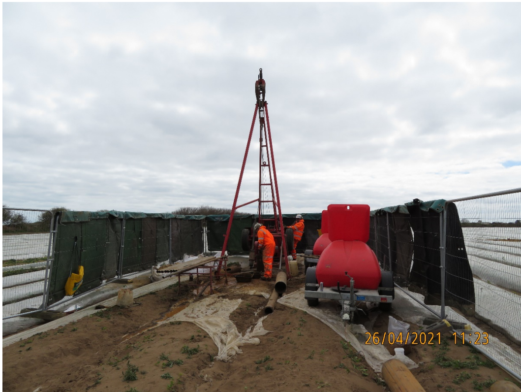
Plate 2.2: Cable Percussion Drilling Rig in Operation at the Landfall
