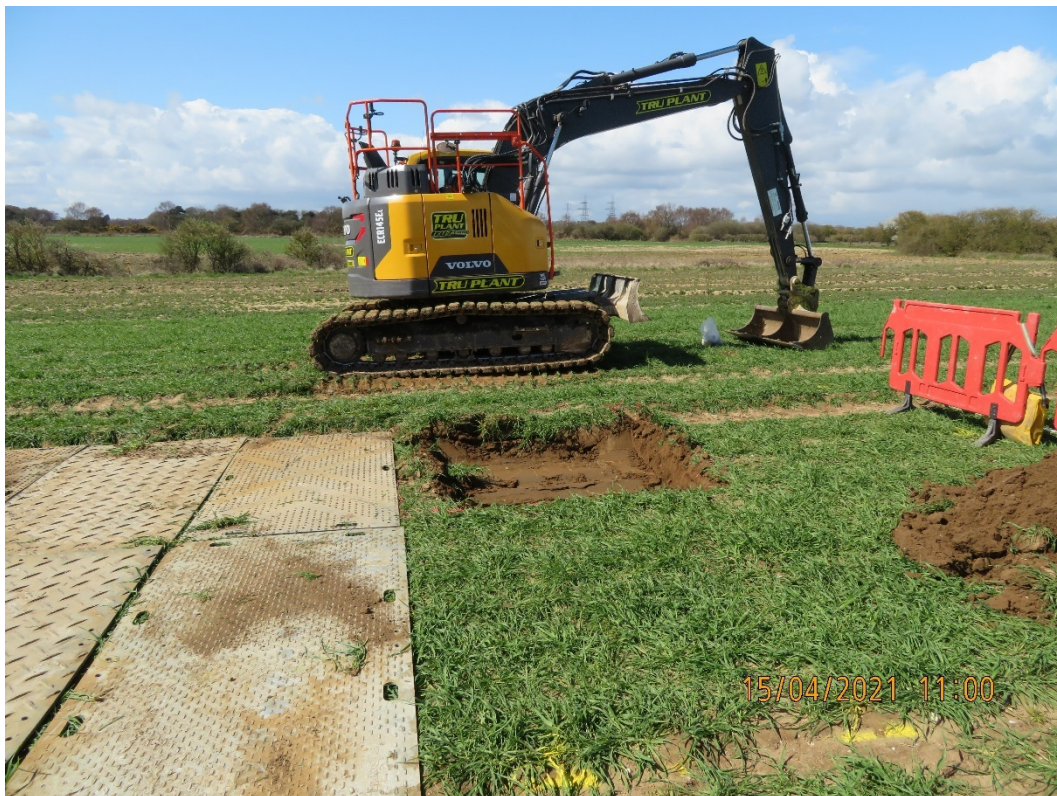
Plate 2.1: Trial Pit Excavation at Onshore Cable Corridor
