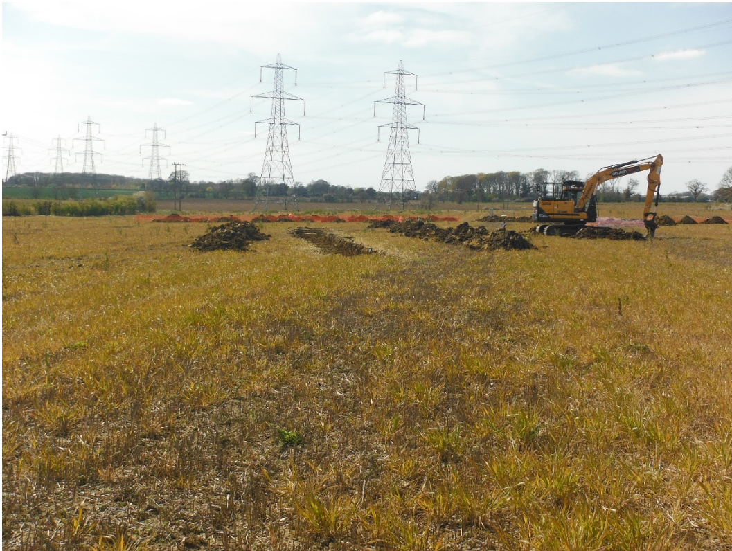
Plate 2.4: Trial Trench Under Excavated at the Onshore Substation Location
